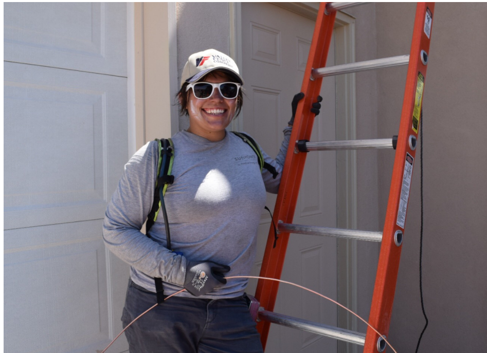
PHOTO: Rita, Solar Installer In New Mexico
